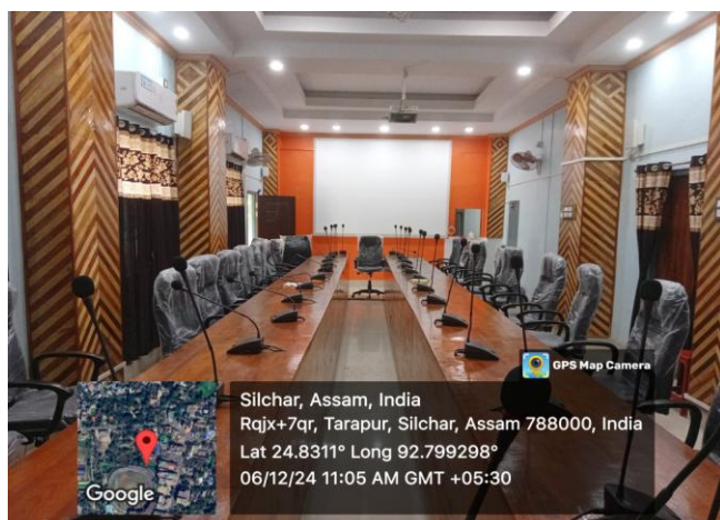
Overhead projector installed in the Conference Hall
